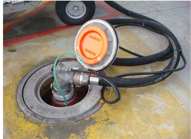
Hydrant coupler and aircraft fueling nozzle swivel retention devices must be equipped with at least two levels of redundancy, such as collar lock rings and collar retention screws secured by safety wire.
